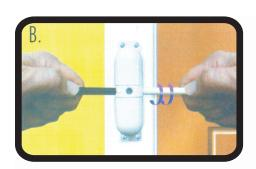
B. Turn the centre of the closer in the opposite direction to the arrow to set the tension. Beware of over tensioning as this may cause the door or gate to slam causing injury or may damage the spring.
